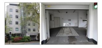
placed in one of the 19 spaces. Retrieval is via another swipe of the key fob at the reader located in the building lobby. A turntable (just visible in the photograph below) ensures that the vehicle is facing the correct way to exit the car park.
