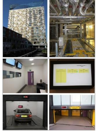
their unit and does not collect it within a given time period, the system re-parks the vehicle so that the lifts are not tied up with un-collected vehicles.
